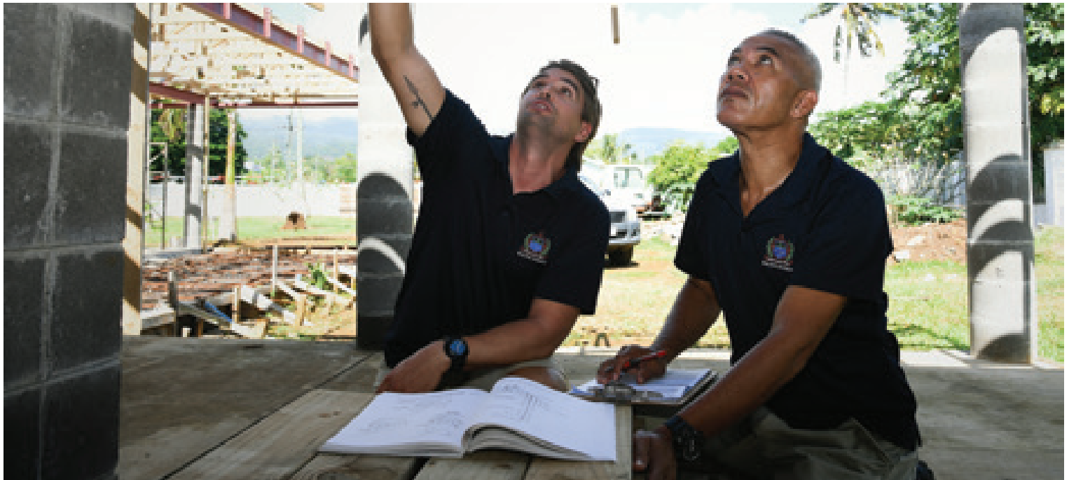
Samoa Australian volunteer Matthew Whitwell (left) and his colleague Joseph Faamatuainu inspecting a new construction. Matthew and Joseph were both engineers with the Ministry of Works, Transport and Infrastructure.
